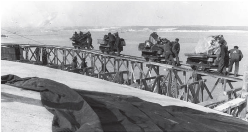
Workers moving granite along the harbour face of the battery, circa. 1916 (PHOTO: CFJIC RE 84-179, from Sarty and Ellis, 2009)
