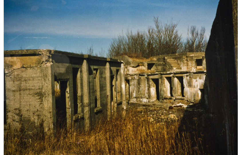
Deteriorating military buildings around battery (PHOTO: J. Doucet)
